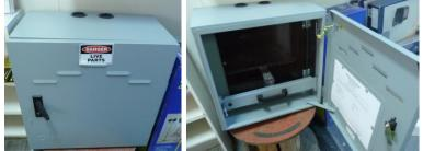
METER ENCLOSURE WITH HINGED PANEL CONTAINING SPACE TO SUIT MAXIMUM OF 2 METER POSITIONS
